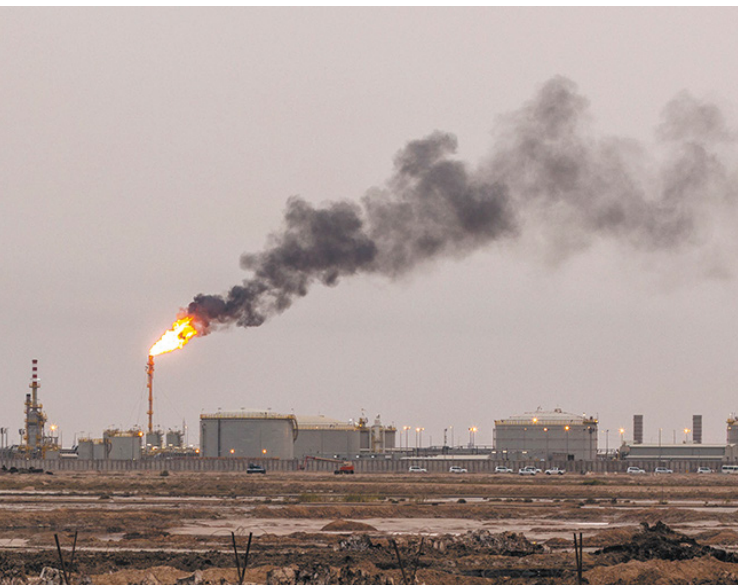
Left: Oil refineries in Kuwait.
