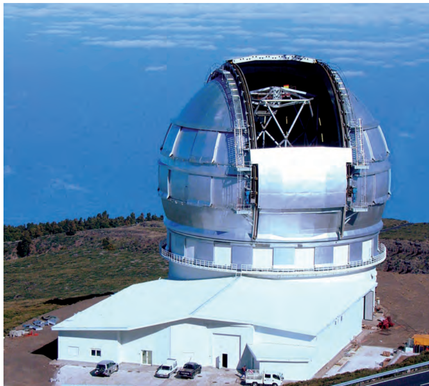
Figure 6. An outside view of the Gran Telescopio CANARIAS (GTC) at the Roque de los Muchachos Observatory of the Canary Islands' Astrophysical Institute. This is the largest and most advanced optical-infrared telescope in the world, with a segmented primary mirror of 10.4 meters in diameter. The low incidence of clouds—the ones visible in this image are actually below the telescope, although the photo's perspective does not make this clear—along with the transparency and stability of its atmosphere make this one of the extremely rare places on Earth where such an advanced telescope can be profitably installed. A large lens, excellent optics and powerful focal instrumentation, as well as the extraordinary astronomic quality of the sky over La Palma, make the GTC an extremely powerful tool for penetrating the secrets of the universe. IAC.
