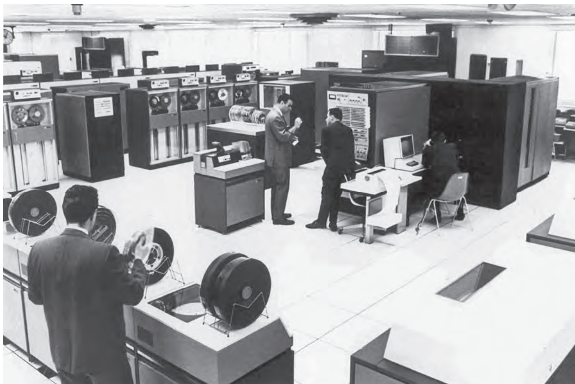
IBM System 360 Mainframe Installation, ca. 1965. The System 360 was one of the most popular and influential mainframe computers, and formed the basis for IBM's main line of business into the 1990s. Smithsonian Institution.
